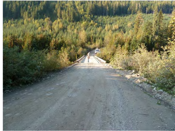
Figure 1-2: Looking towards woods end.
