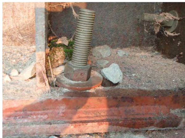
Figure 1-12: Slotted plate and bent anchor bolt on camp end downstream corner.
