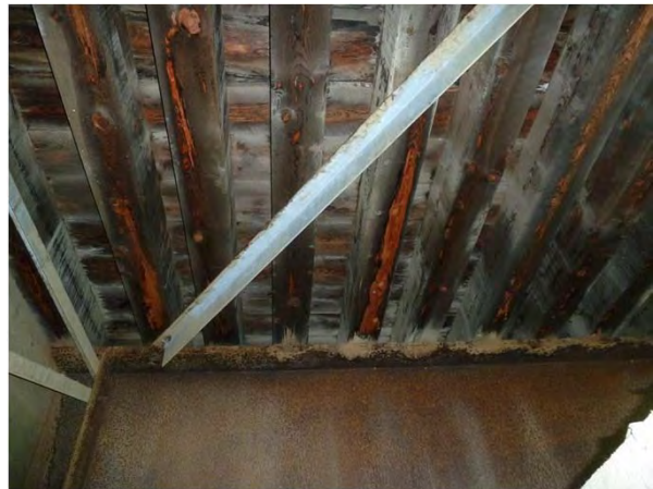
Figure 1-8: Typical condition of underside of deck.
