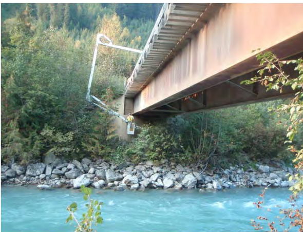
Figure 1-15: Woods end abutment.
