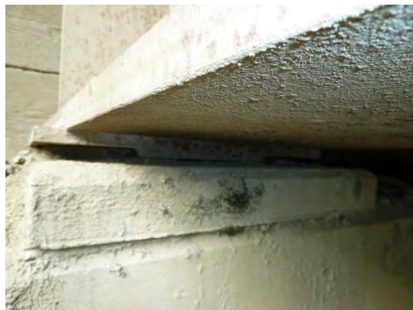
Figure 1-18: Woods end downstream bearing.
