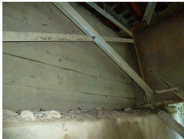
Figure 1-16: Woods end ballast wall.
