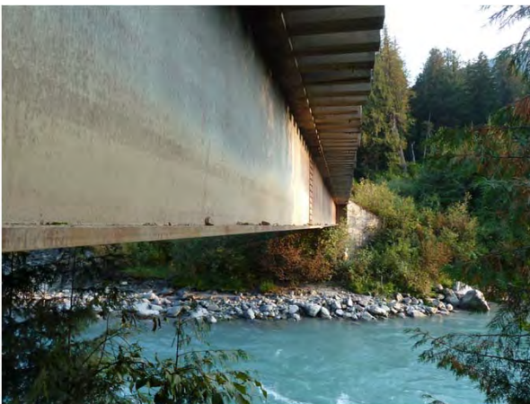
Figure 1-9: Downstream face looking towards camp end.
