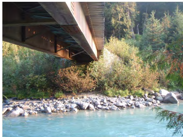
Figure 1-10: Camp end abutment.
